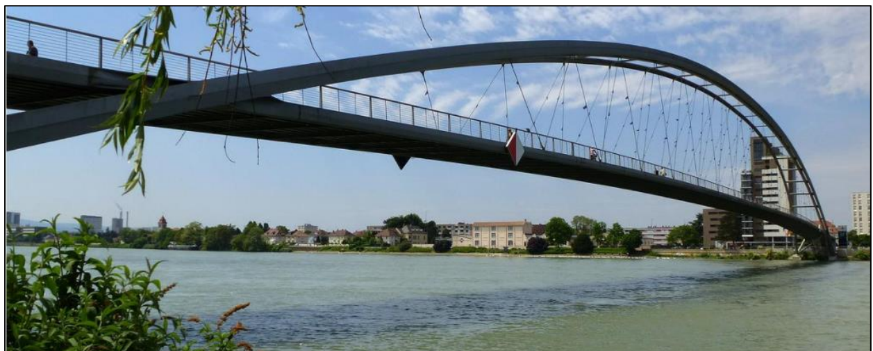
Figure 3. “Three Countries Bridge” single-span bridge dedicated to pedestrians and cyclists
