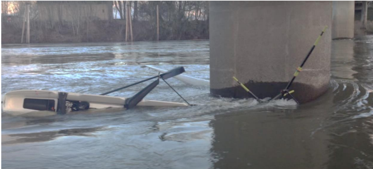
Figure 1. Example of bridge pier impact by rowing boat and current effects
